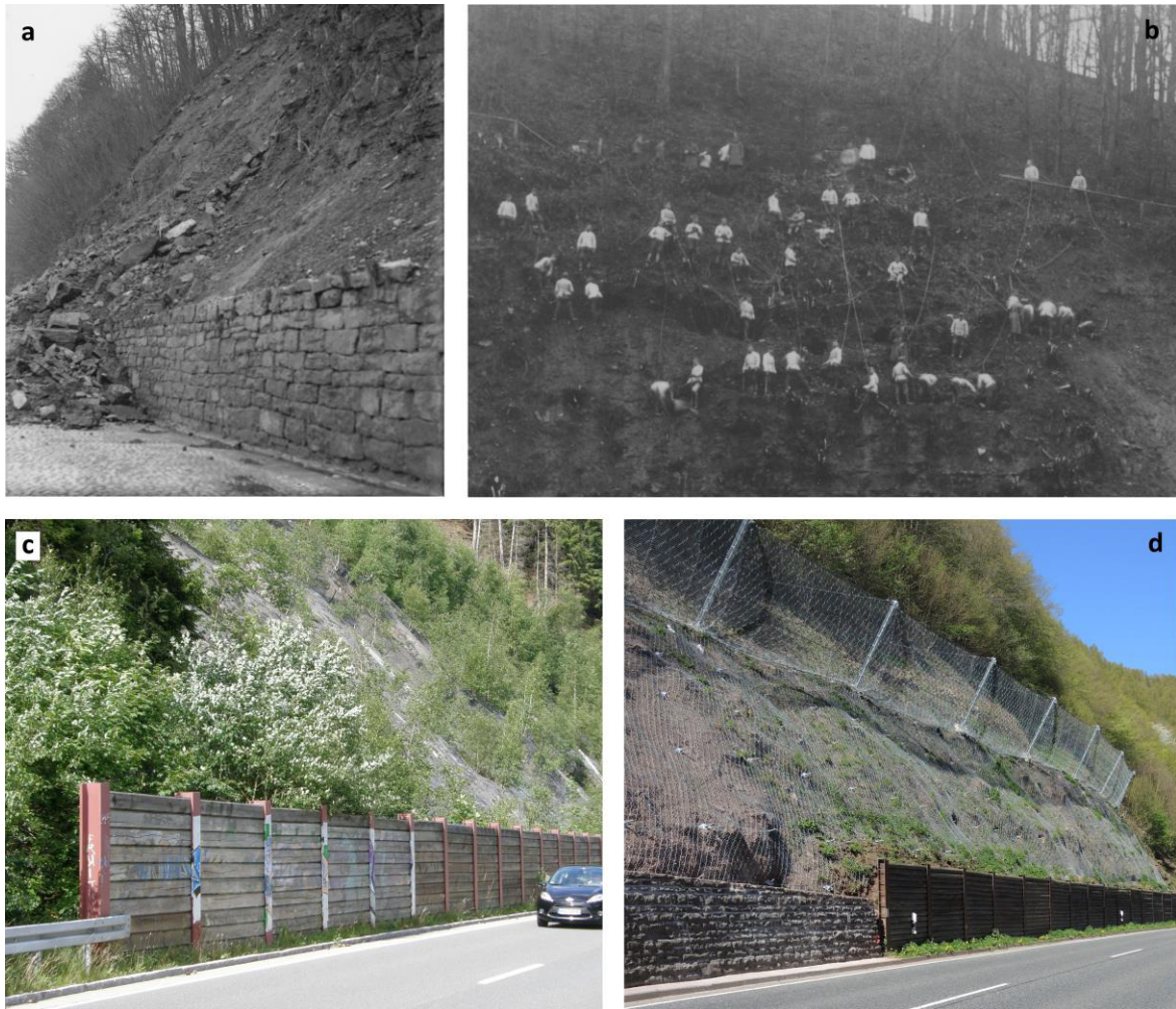
Figure 19. Development of mitigation measures in southern Lower Saxony, NW Germany. (a) The drywall construction from the 1930s in the front did not contribute to protection against rockfalls/slides. (b) Removal of loose rock and vegetation in the Upper Weser area in 1936. (c) Combination of steel buttress/wooden planks as a barrier against rockfall on an interstate road in the Harz Mountains, NW Germany. (d) Rockfall mitigation in the Upper Weser area. The barrier wall in the left and wooden barrier in the right foreground are constructed in 1983, rock drapery and catch fence constructed in 2015.
